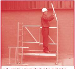
5. If required (see component table on back page) add an extension frame by locating the conical fittings of the extension frame into the top of the end frame of the folding unit ensuring that the pegs engage in the holes provided.
