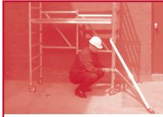
7. Locate guardrail brace(s) 4 rungs above the rung on which the platform will be located ensuring that the brace hooks clip onto the frame uprights above the rung with the spring loaded pin facing outwards. Double guard railing can be achieved by locating 2 additional guardrail braces 2 rungs above the platform position. Relocate the platform to its final location and if working outdoors secure the wind latch underneath the platform
