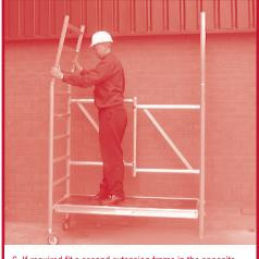
6. If required fit a second extension frame in the opposite end frame engaging the conical fittings in the same manner
