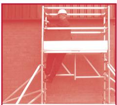
9. Always gain access to the platform by climbing up the rungs on the inside of the unit and gaining access to the platform through the trap door provided. Always shut the trap door immediately after climbing through. If required an Alto M.D. tower folding toe board can be fitted.
