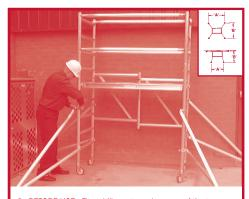
8. BEFORE USE: Fit stabilisers to each corner of the tower to increase the effective base dimension "A" & "B". They must be fitted so that when viewed from above, the largest square is formed. Ensure that the wing nuts are tight so that it is not possible to move the stabilisers without slackening the wing nuts. Do not overtighten them as this may distort the tube.
